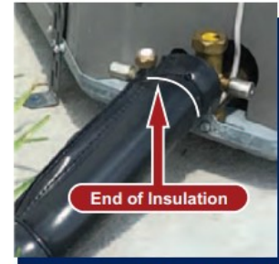
Pipe-Insulation Ends Must Be Protected
