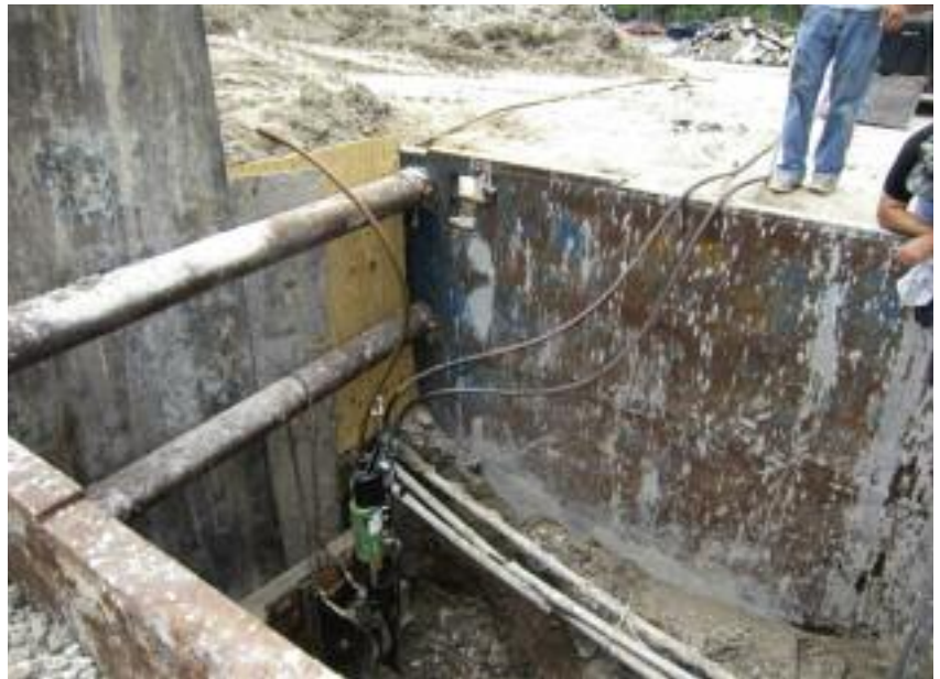
A 100 Ton Ram Winch Pulling New HDPE Pipeline 270'
