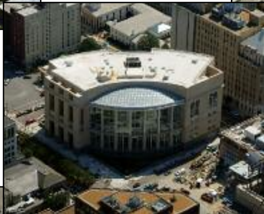
Richmond Federal Courthouse
